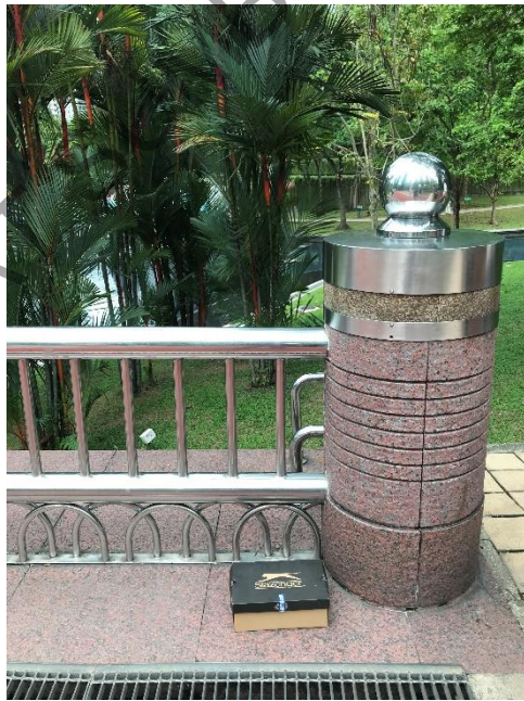
Figure 3.11 Bridge in the KLCC Park
