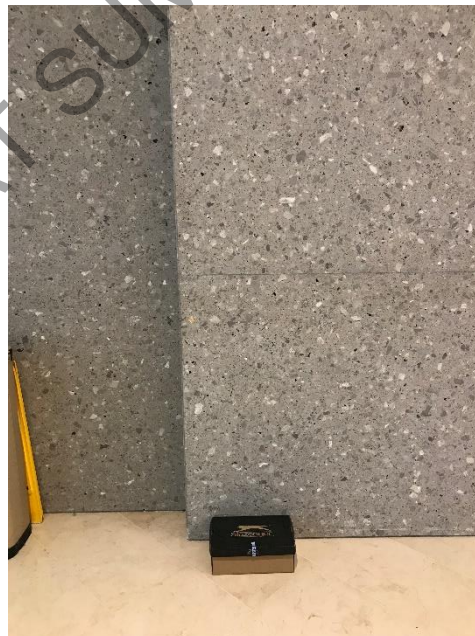
Figure 3.5 Ground Floor of Suria KLCC (West)
